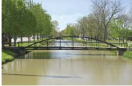
1864 Cast Iron Bridge is the oldest bowstring girder bridge in Ohio.
