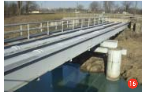
The Aqueduct as seen today
